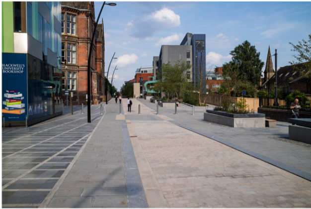
New combined cycleways & servicing routes at the University of Sheffield
