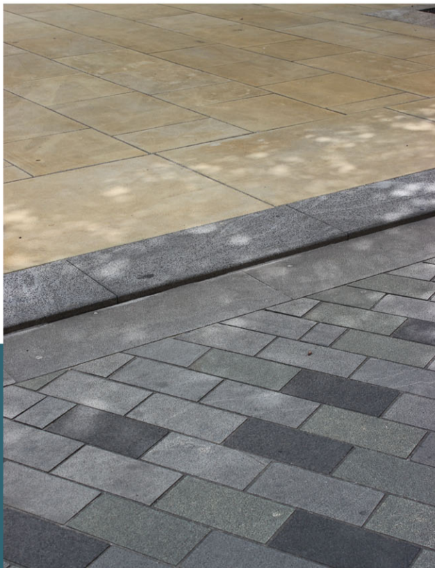
Provide sandstone footways & granite surfaces on heavily used routes, that also helps to define cycling & servicing areas
